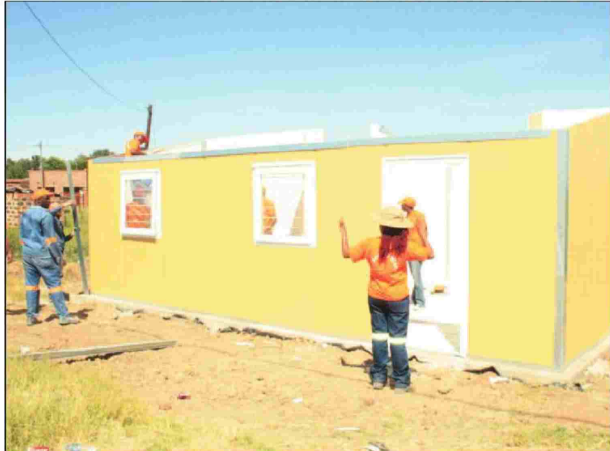
One of the houses which are near completion in Blaauwbosch
